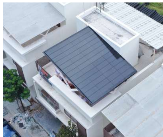
Fig. 4.7 . Aerial view of the PowerRoof. Source: SunEdison
