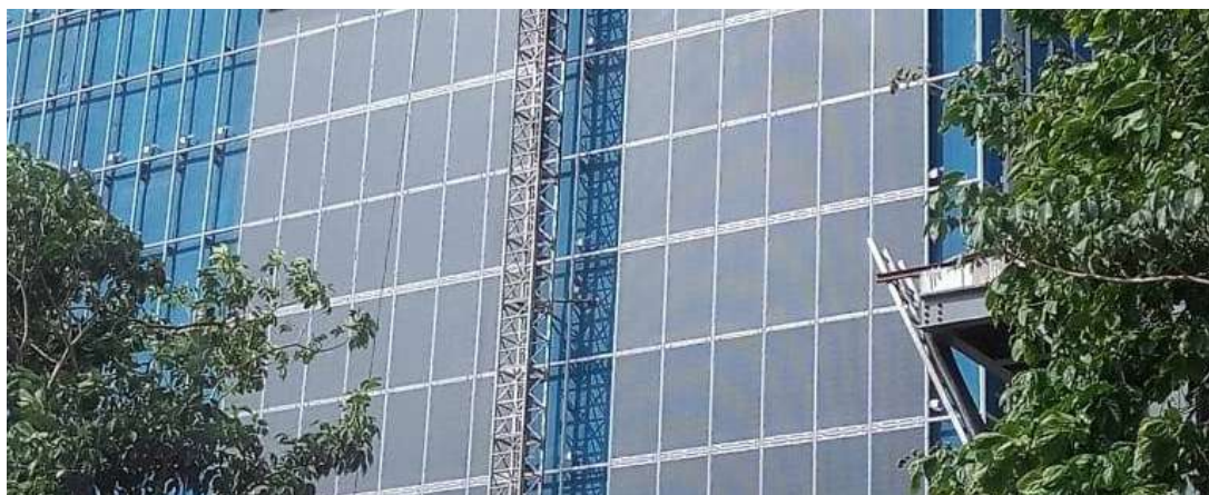
Fig. 4.3 CTRLS during the BIPV facade construction phase. Source: U-Solar.
