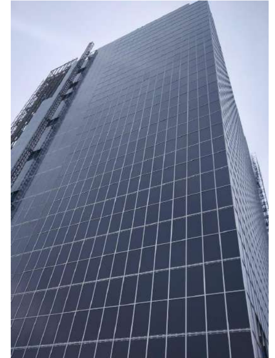
Fig. 4.4 CTRLS BPV facade. Source: U-Solar.
