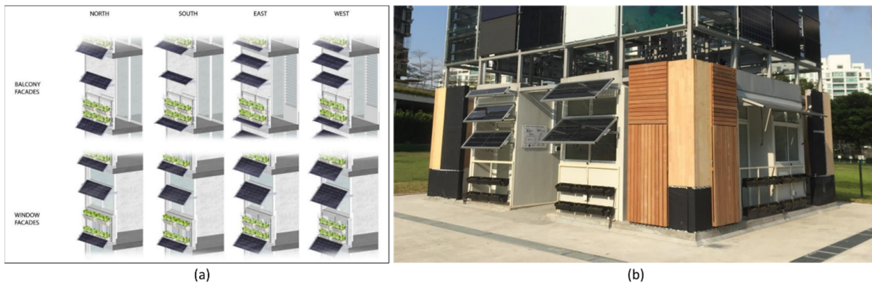
Figure 8. (a) Eight PF prototypes under four orientations; (b): Photograph of the constructed PF at the NUS T2 Lab [92].
