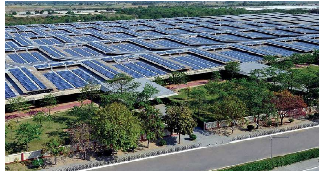
Fig. 1.12 RSSB-EES in Beas. Source: L&T Construction.
