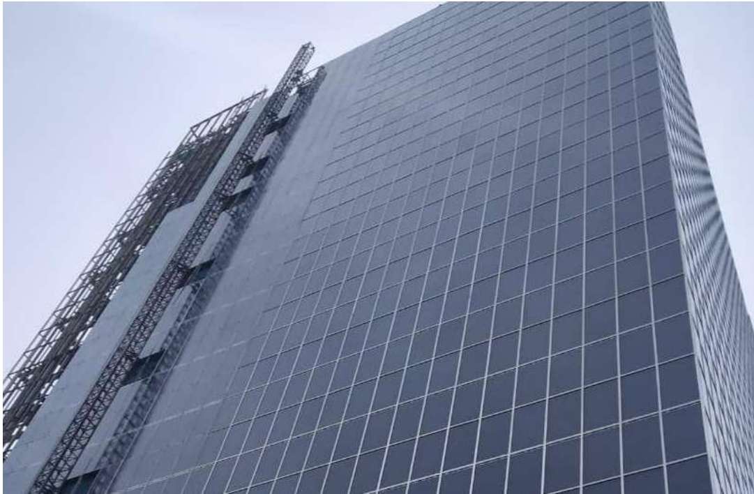
Fig. 1.13 CTRLS Data Center, Mumbai. Source: U-Solar.
