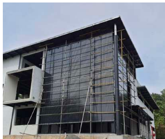
Fig. 4.11 Curtain wall under construction. Source: TopSun
